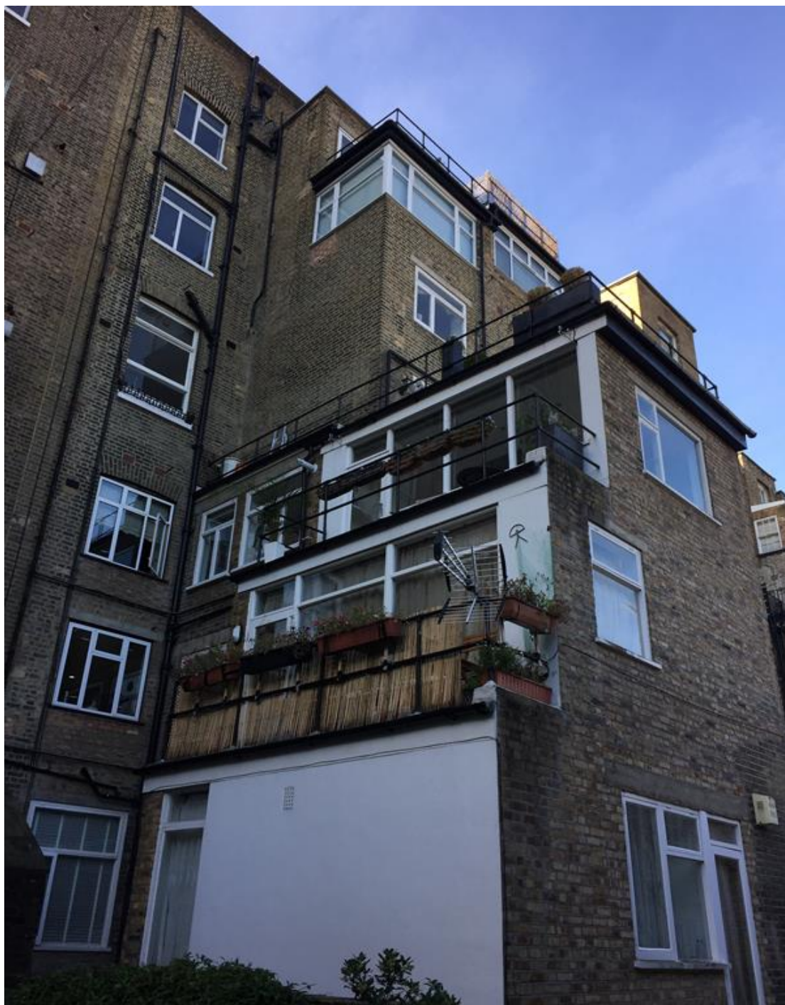
Rear elevation of Flat M 9-11 Westbourne Terrace
